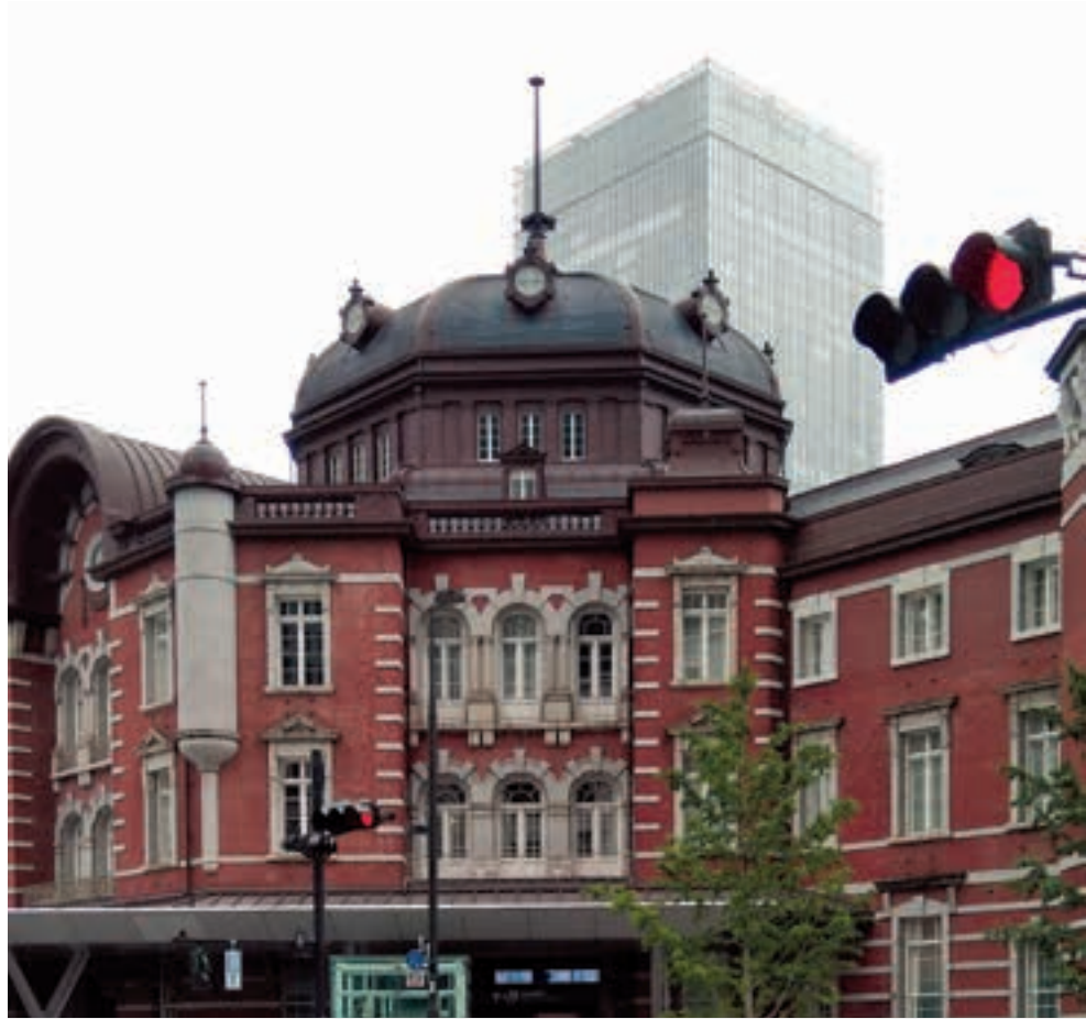
Tokyo Railway Station
